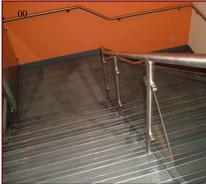
Haiku Carpet Tiles fitted to Stairs and landings, including Gradus Aluminium Stair Nosings
