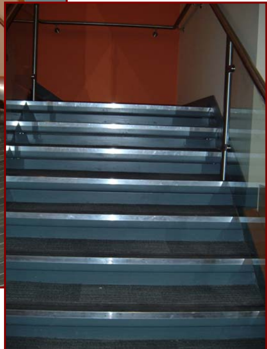
Haiku Carpet Tiles fitted to Stairs and landings, including Gradus Aluminium Stair Nosings
